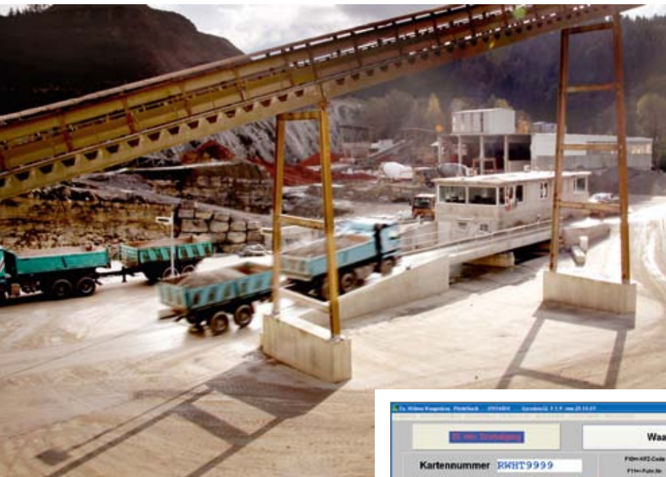
Central Control Room with entry/exit scale
